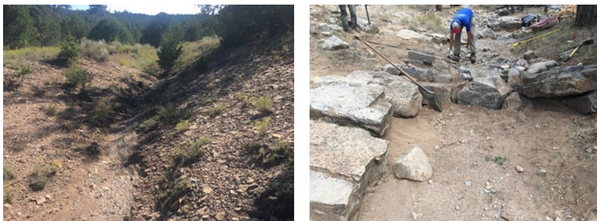
Figure 5. Bank erosion (left) and structure installation (right). Photo credit: Rocky Mountain Youth Corps/Stream Dynamics, 2019
