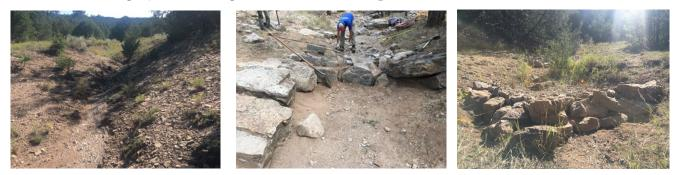
Figure 15. Bank erosion (left), structure installation (center), and installed structures (right). Photo credit: Rocky Mountain Youth Corps/Stream Dynamics, 2019
