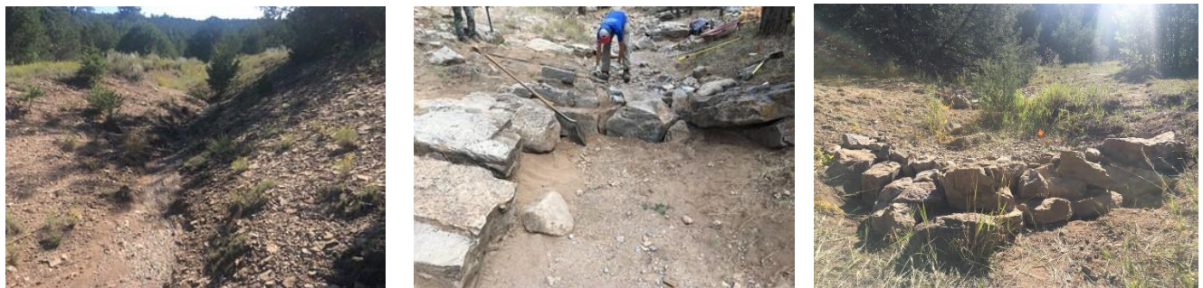
Figure 15. Bank erosion (left), structure installation (center), and installed structures (right).
